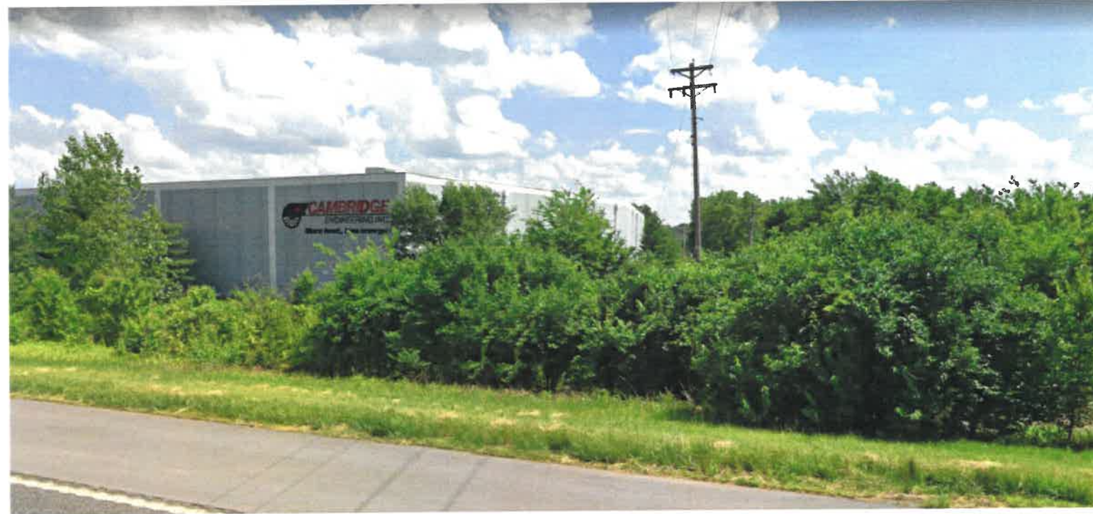
EXISTING NORTHWEST BUILDING CORNER VIEW
