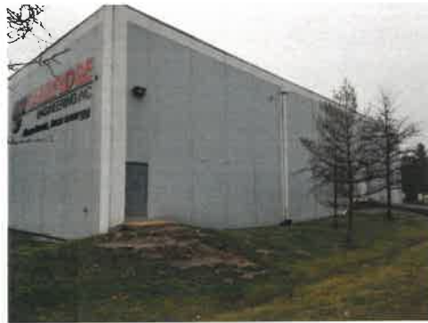
PHOTO #7 LOOKING NORTHWEST CORNER OF BUILDING
