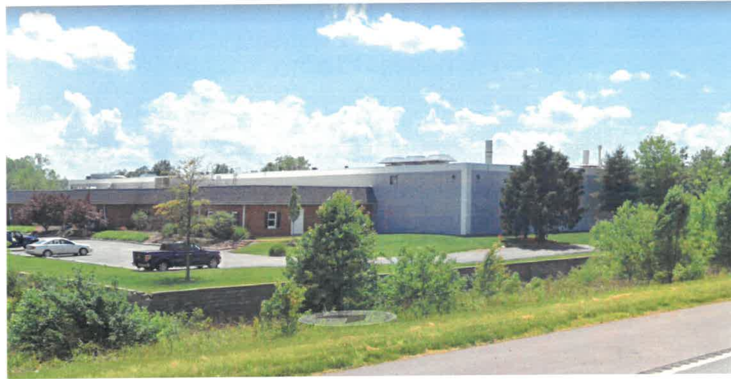
EXISTING NORTHEAST BUILDING CORNER VIEW
