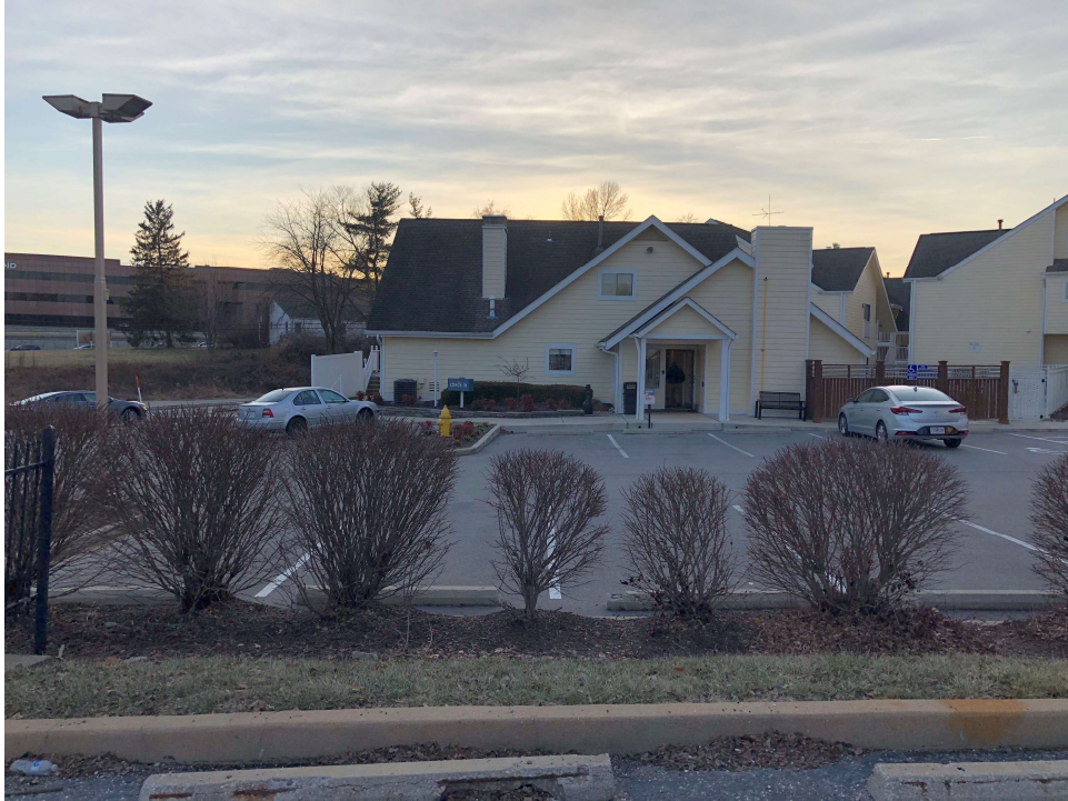
Looking towards property to south
