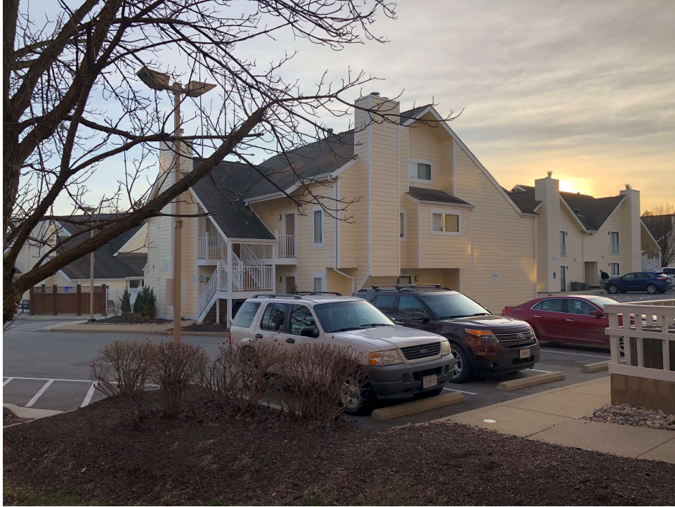
Looking towards property to south
