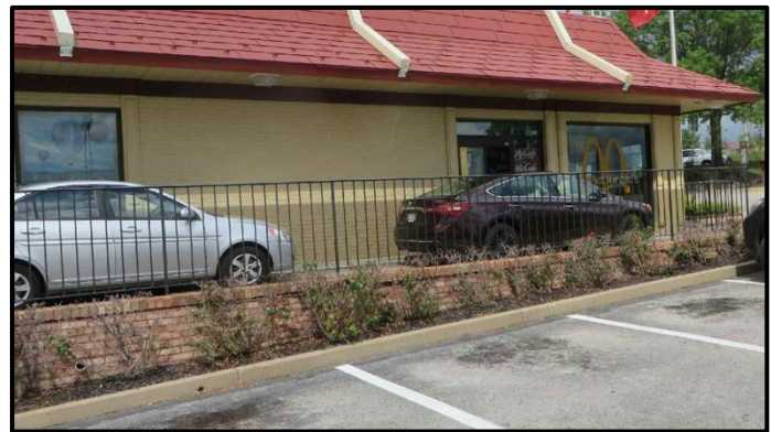
Figure 6: Existing Retaining Wall to Remain
