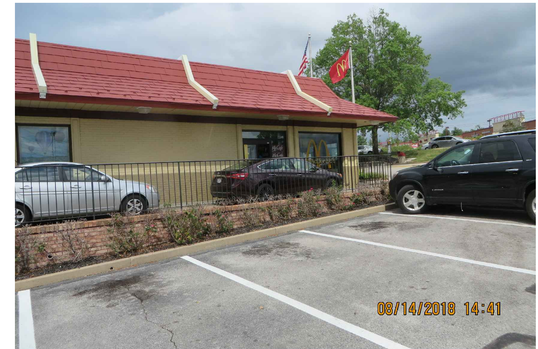
EXISTING RETAINING WALL ALONG DRIVE THRU SIDE - REAR SIMILAR
