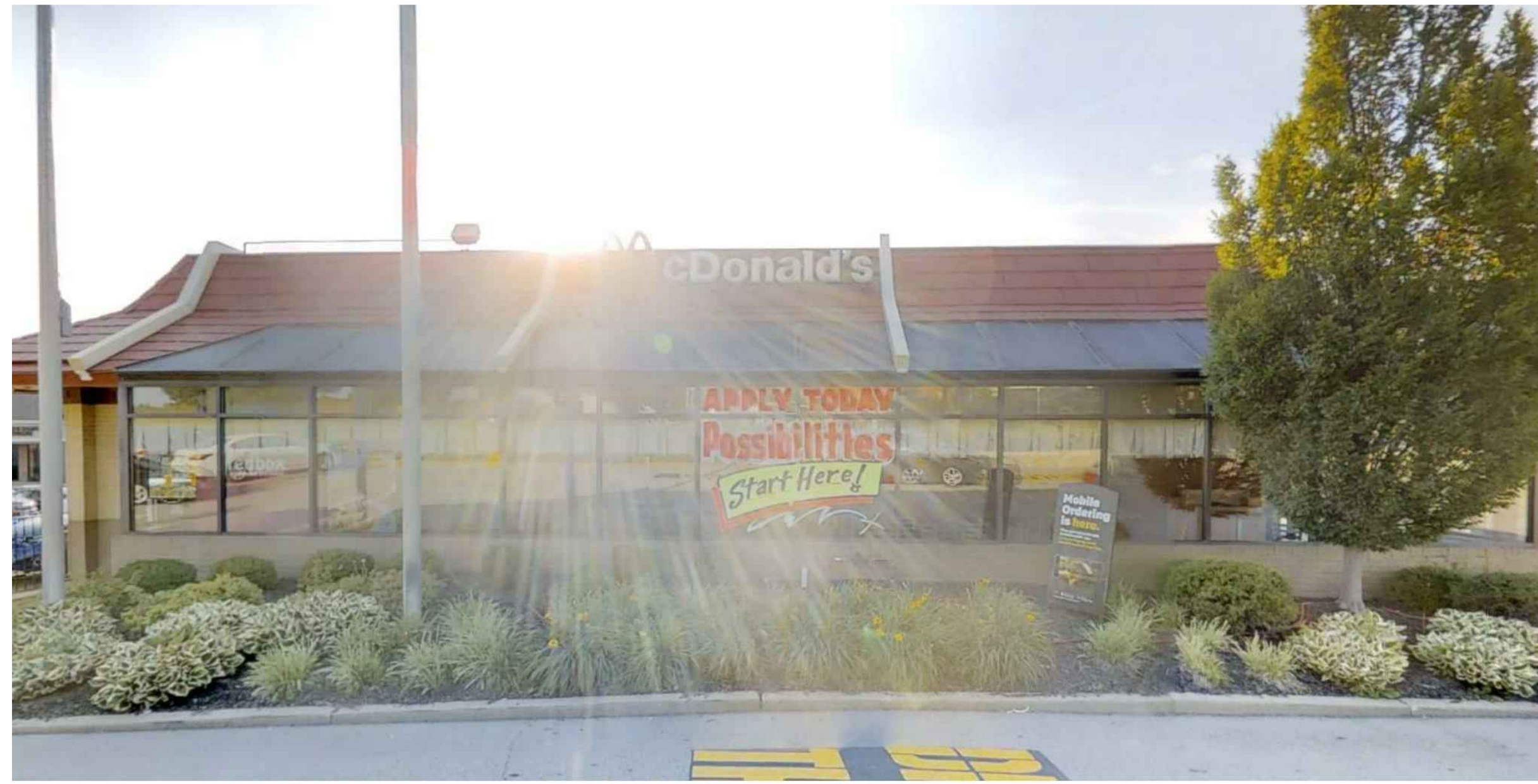
EXISTING BUILDING FRONT ELEVATION
