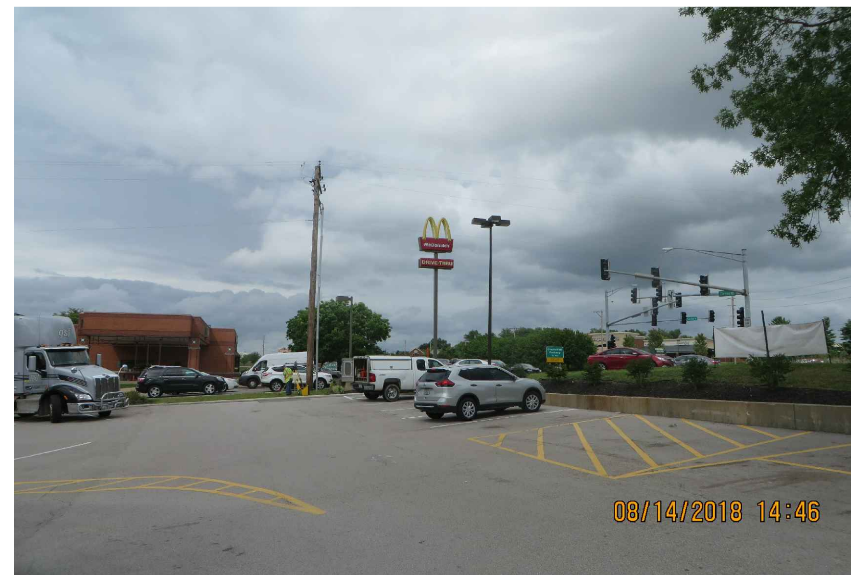
EXISTING CONCRETE RETAINING WALL ALONG SITE FRONTAGE
