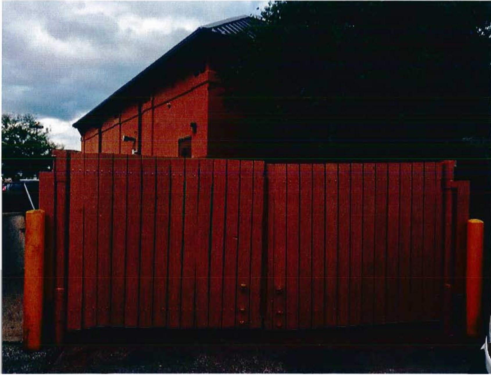
View of the existing trash enclosure from the southwest
