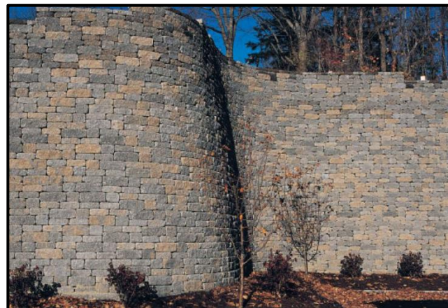
Figure 5: Mosaic Retaining Wall
