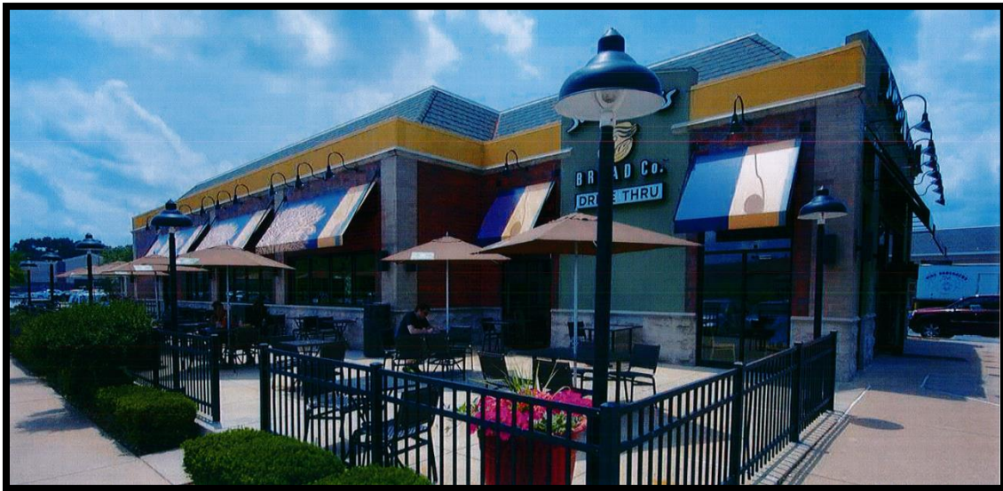
Figure 2. Existing Conditions of East Elevation
