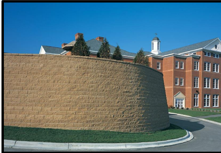
Figure 4: Retaining Wall Material image
