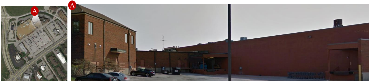
Rooftop Equipment of Building D as seen from Hilltown Village Ctr. Right-of-Way
