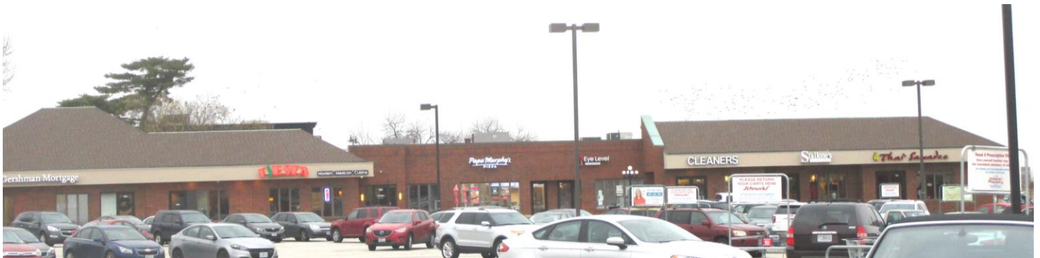
Existing Building A
