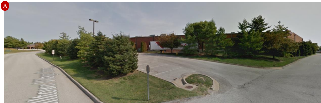
Rooftop Equipment of Building C as seen from Right of Way
