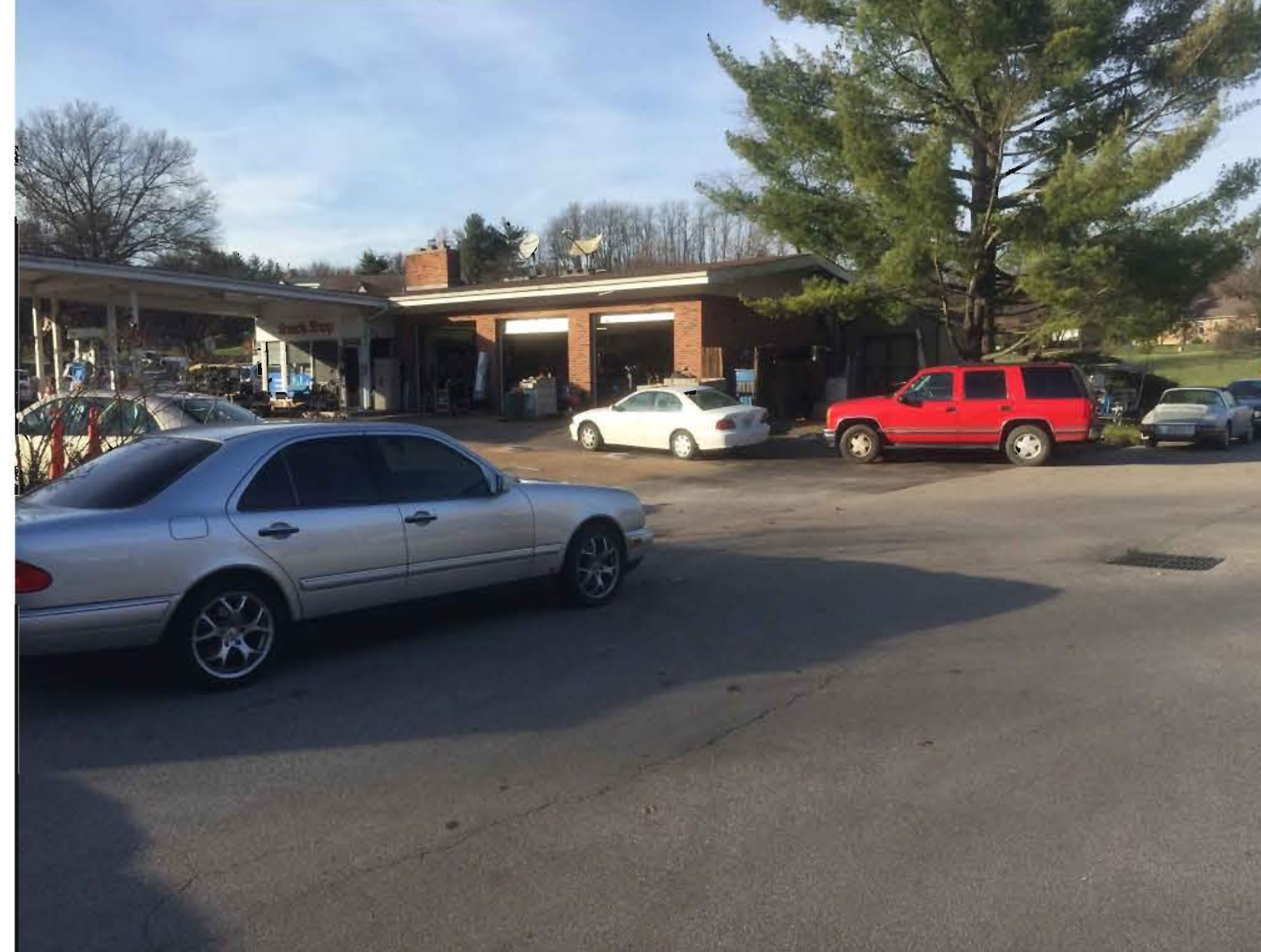
LOT A2 NORTHWEST VIEW
