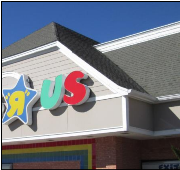
Existing Clipped Gable Roofline
