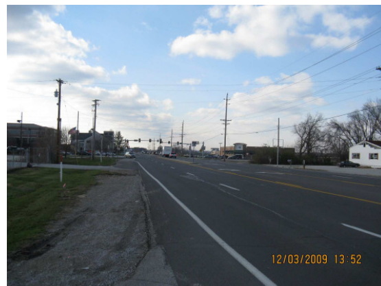
View Looking west along Chesterfield Airport Road.
