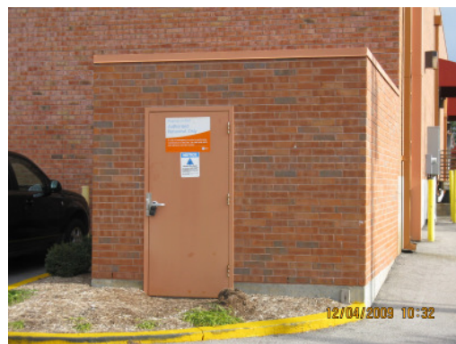
Existing equipment room
