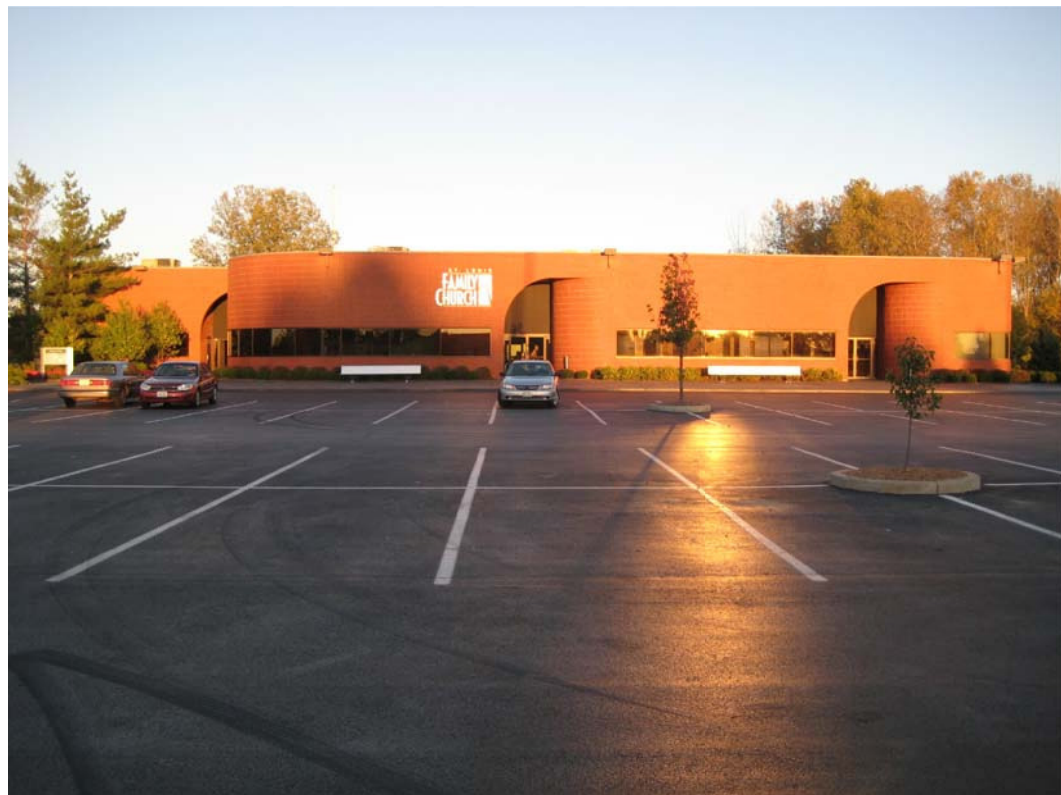
EXISTING SANCTUARY BUILDING - WEST FACADE
