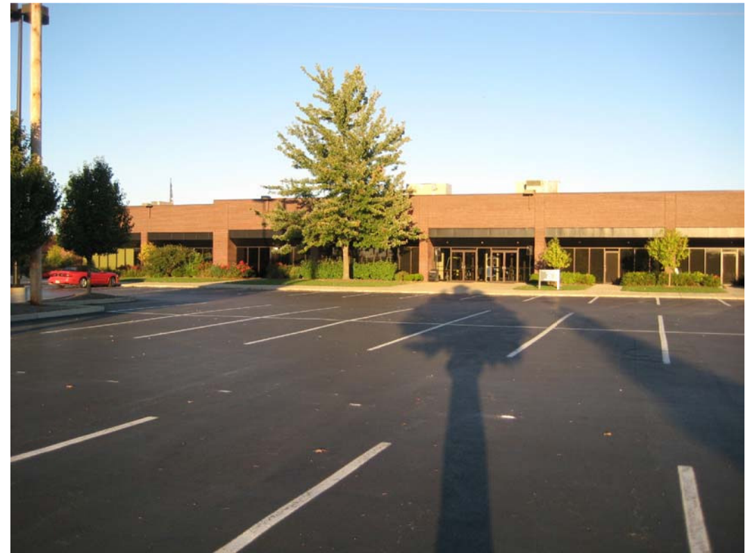
EXISTING YOUTH BUILDING - WEST FACADE
