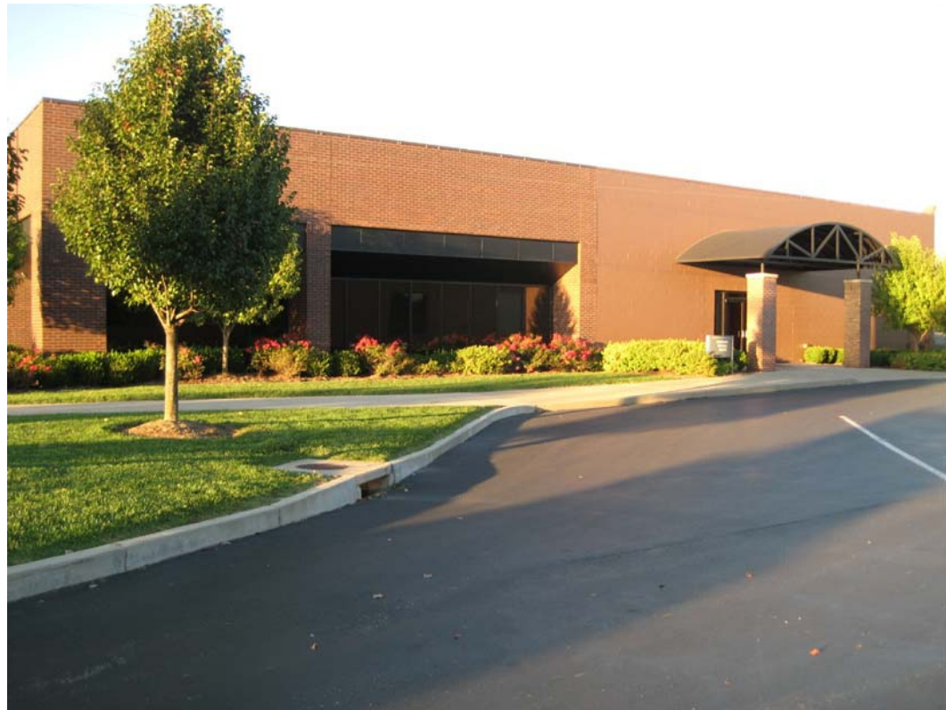
EXISTING YOUTH BUILDING - SOUTH FACADE
