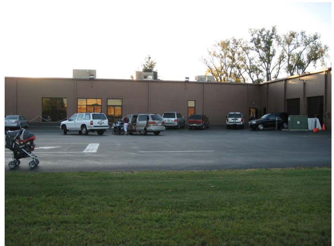
EXISTING YOUTH BUILDING - EAST FACADE
