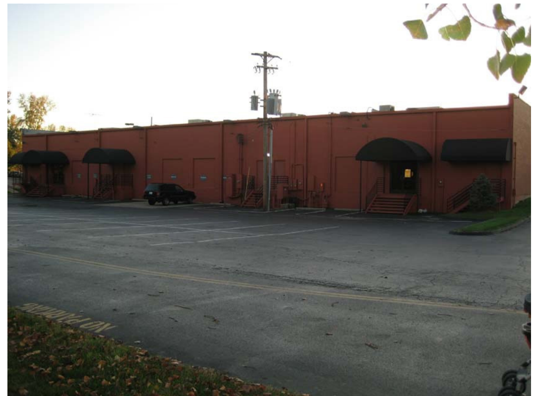
EXISTING SANCTUARY BUILDING - EAST FACADE
