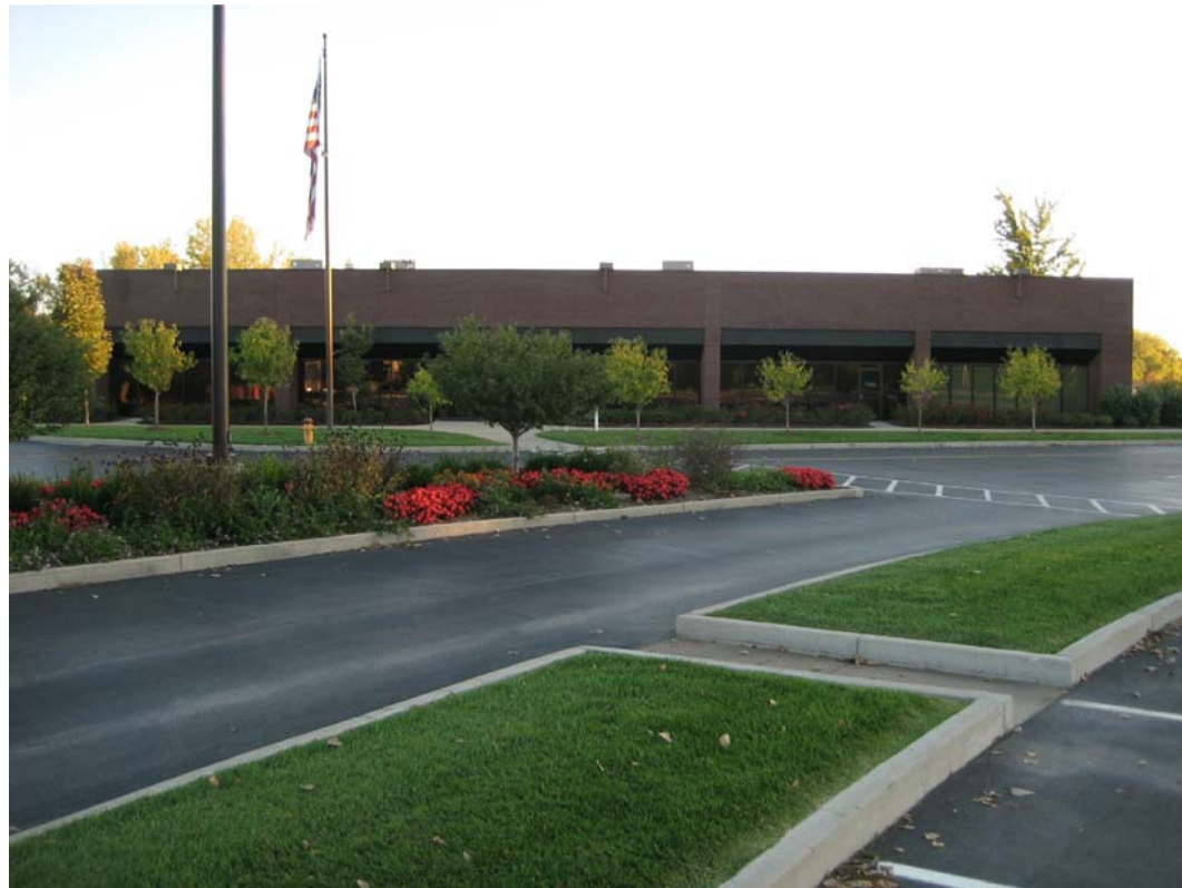
EXISTING YOUTH BUILDING - NORTH FACADE
