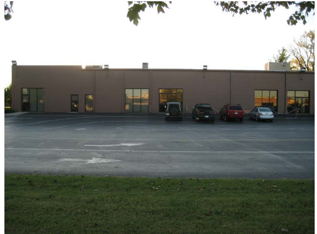
EXISTING YOUTH BUILDING - EAST FACADE
