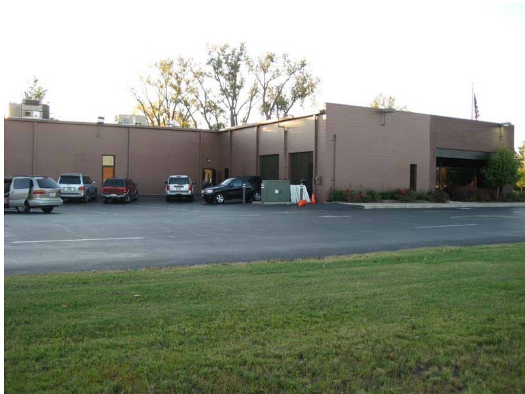
EXISTING YOUTH BUILDING - EAST FACADE
