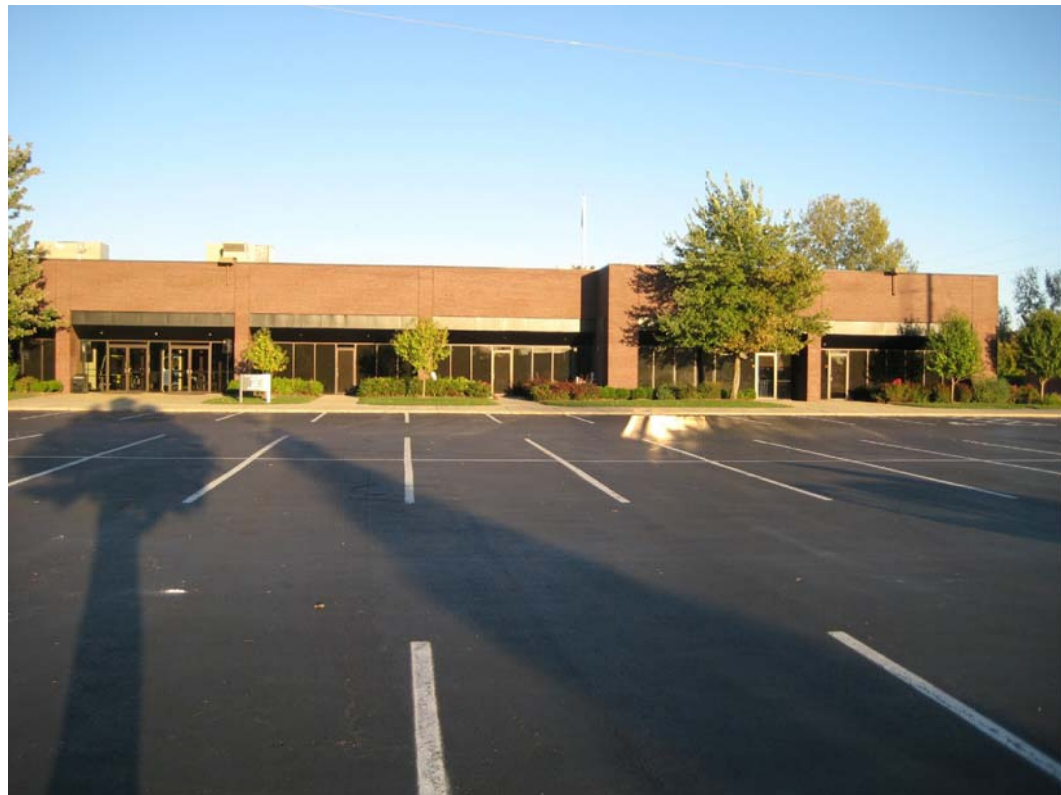
EXISTING YOUTH BUILDING - WEST FACADE
