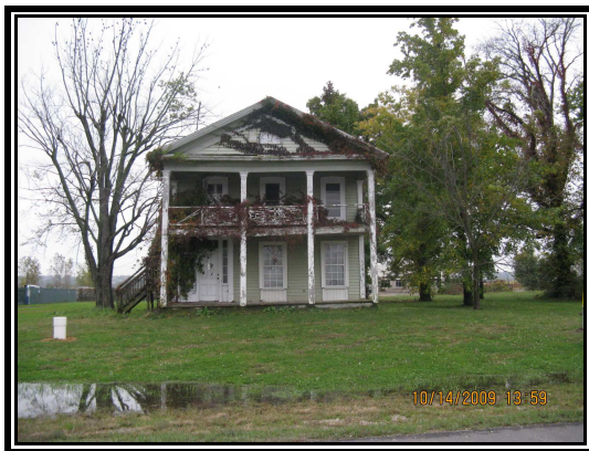
Looking south at the existing residential structure on the site from Olive Street Rd.
