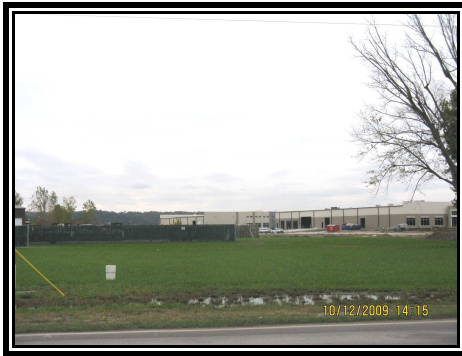
Looking south at the property to the west of the subject site (Spirit Valley Business Park)
