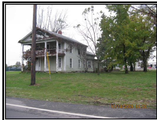
Looking southeast at the existing residential structure on the site from Olive Street Rd.
