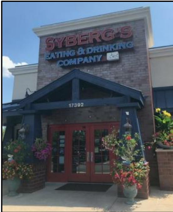
Figure 3.a: Existing Main Entrance
