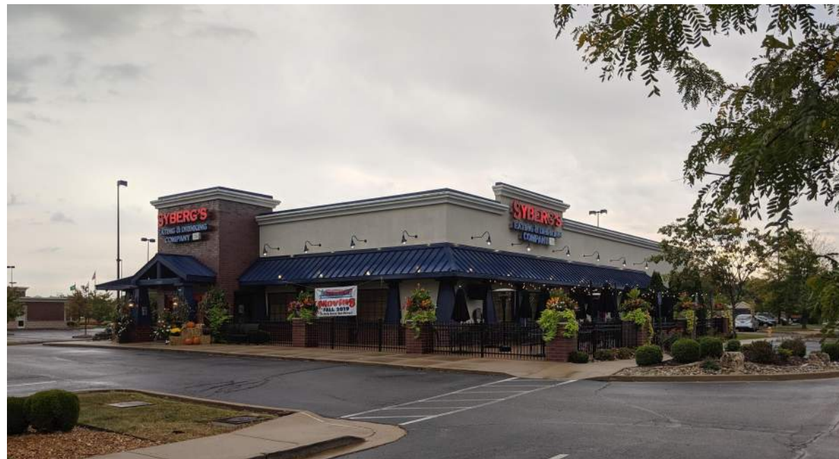
existing nw corner
