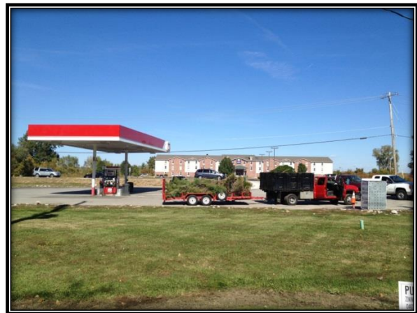
Existing Service Station Canopy—View from Old Olive Street Road
