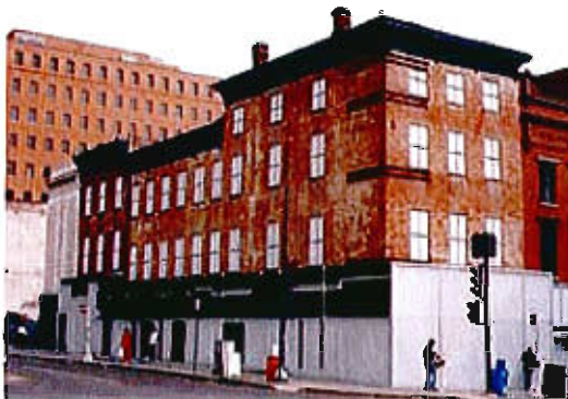
Urban buildings often need additional protection from unwanted entry and graffiti. This commercial building uses painted plywood panels to cover its glass storefronts. The upper windows on the street sides have been painted to resemble 19th century sash. Photo: NPS files.
