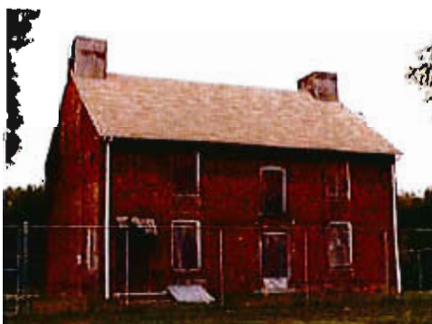
A view showing the exterior of the Brearley House, New Jersey, in its mothballed condition. Photo: Michael Mills, Ford Farewell Mills Gatsch, Architects.
