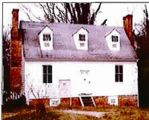
Regrading has protected this masonry foundation wall from excessive damp during its 10-year mothballing. Note the attic and basement vents, temporary stairs, and interpretive sign. Photo: NPS files.
