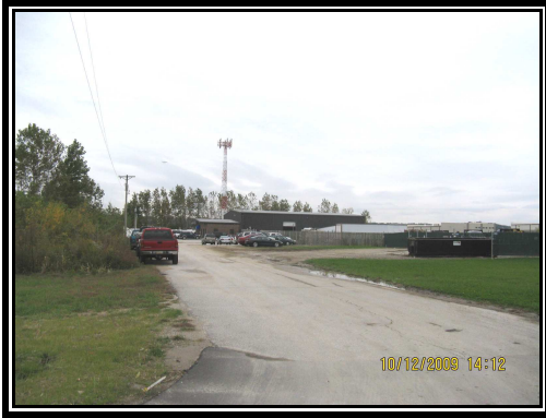
Looking south at the subject site
