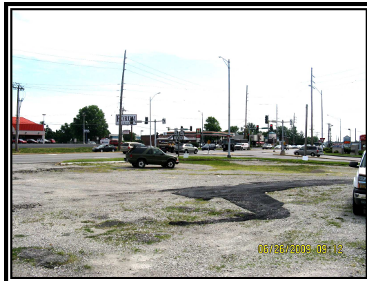
Looking southeast across the subject site
