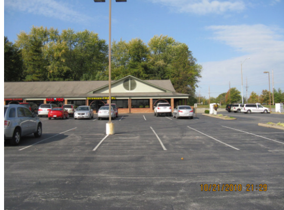
View looking west at the end cap of the existing building
