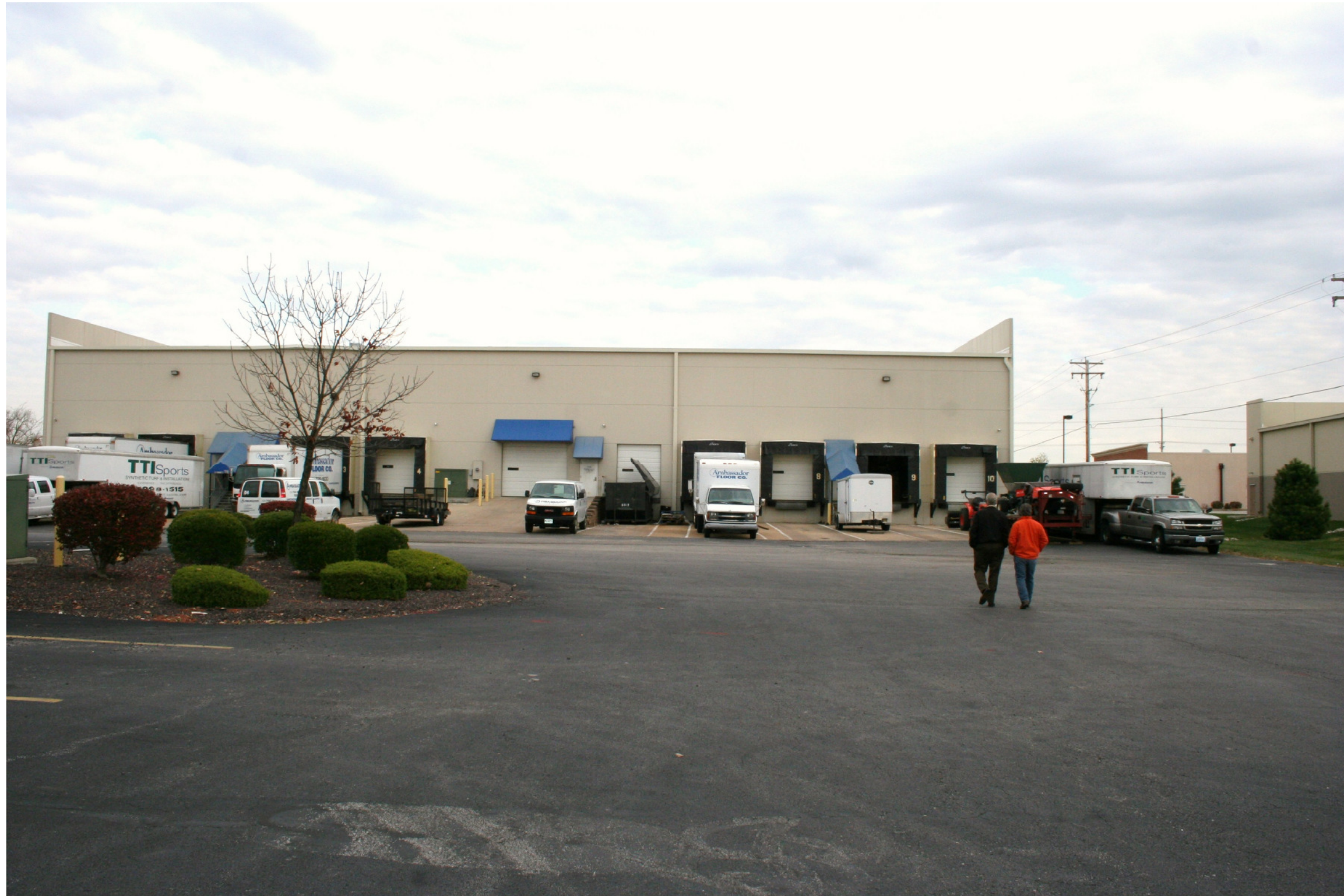
View from center of site looking North
