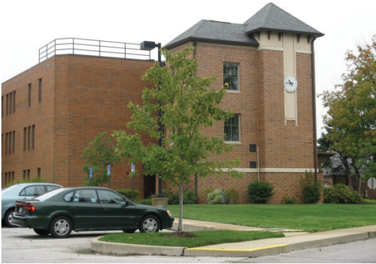
View of the existing multi-story structure on the site
