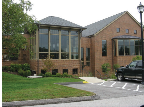
View of the Multi-Purpose addition
