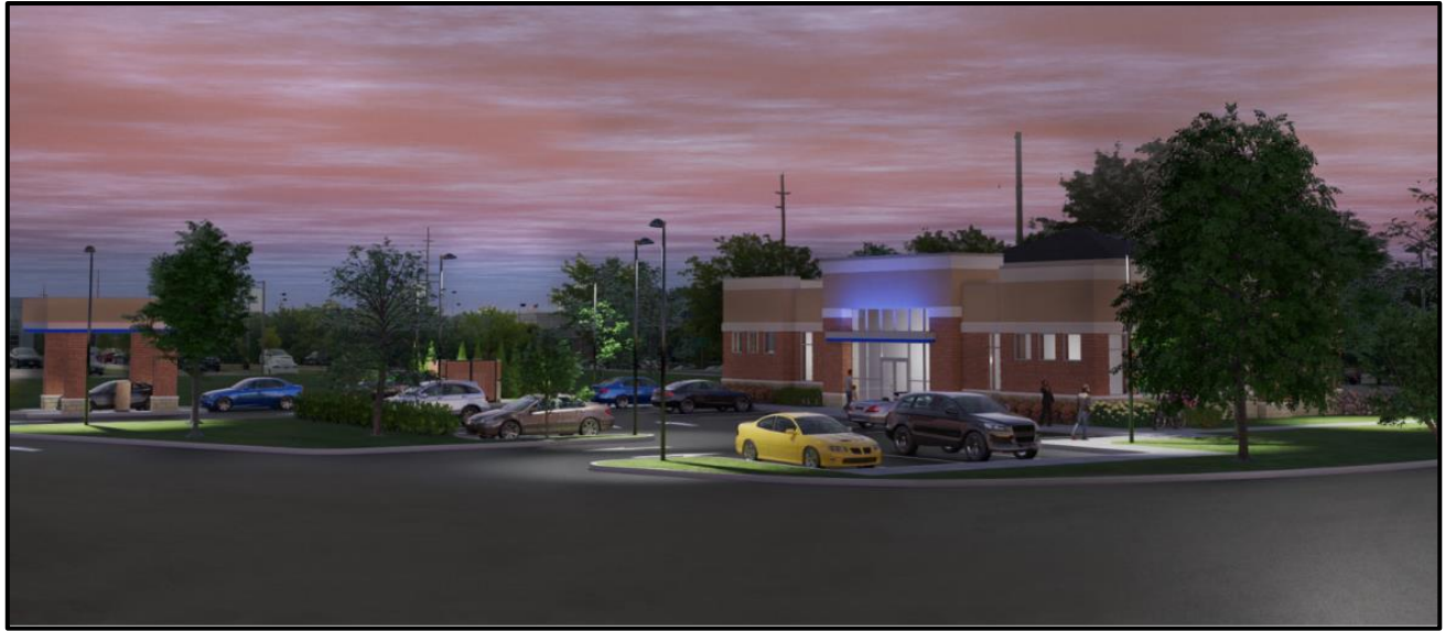
Figure 3: North Elevation as seen from parking lot.
