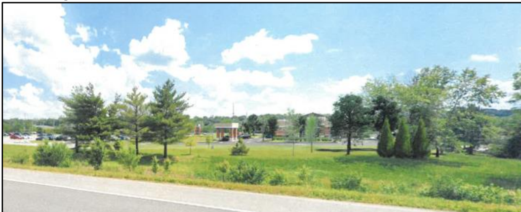
Figure 9: North Elevation as seen by vehicles traveling east on I-64.
