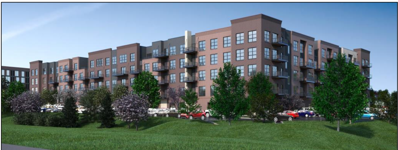
Figure 7: View Heading Southeast on I-64
