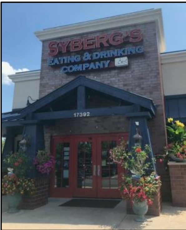
Figure 4.a: Existing Main Entrance
