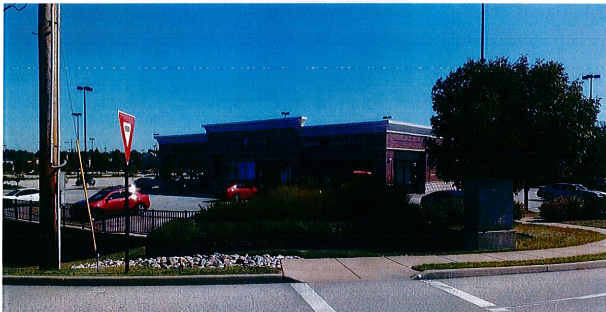
Retail Strip at Southeast Corner of Intersection
