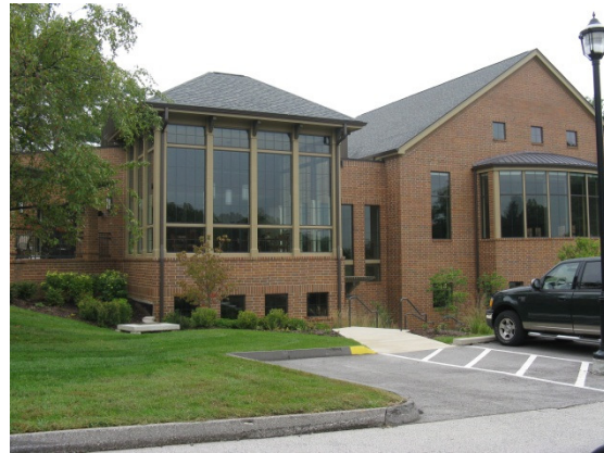
View of the Multi-Purpose addition
