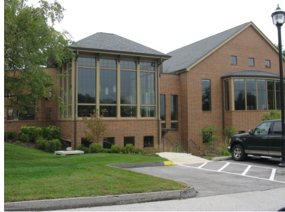
View of the Multi-Purpose addition
