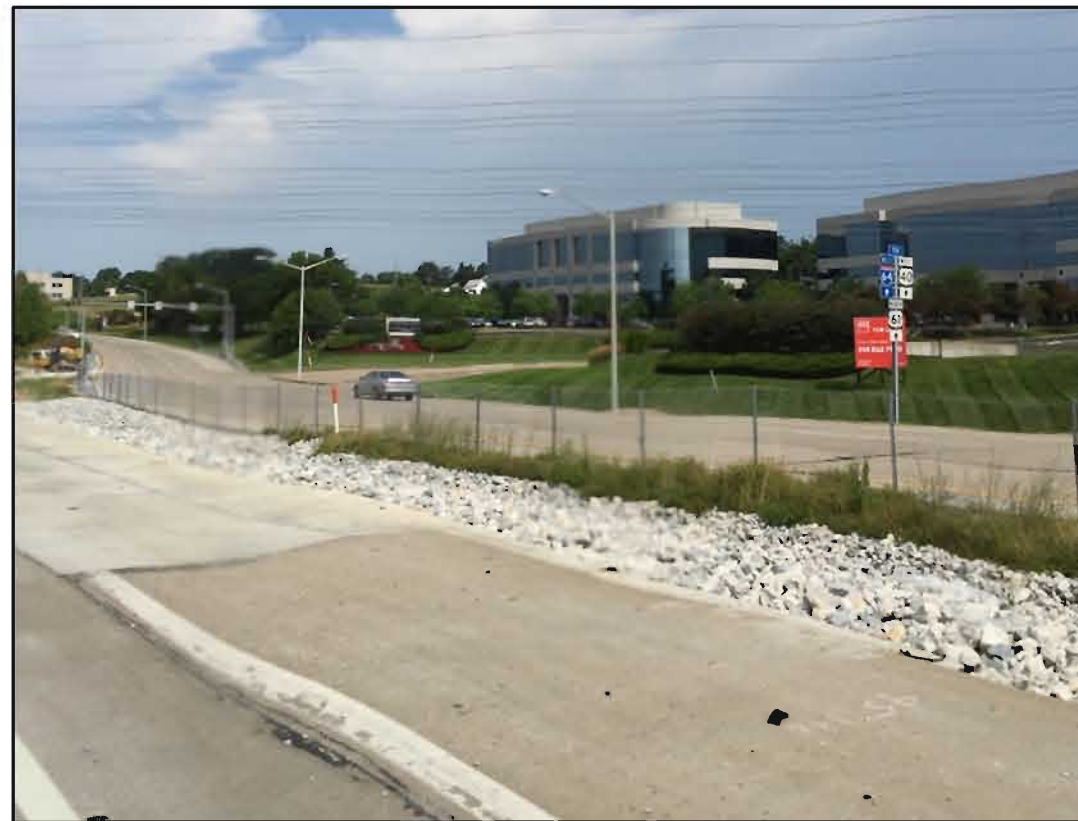
View Looking West Toward Timberlake Corporate Center
