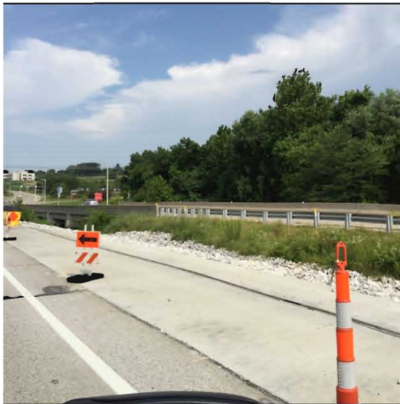
View Looking West Toward Timberlake Corporate Center
