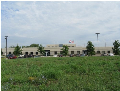
View looking east
