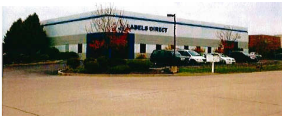
View Looking South East From Entry
