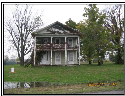
Looking south at the existing residential structure on the site from Olive Street Rd.
