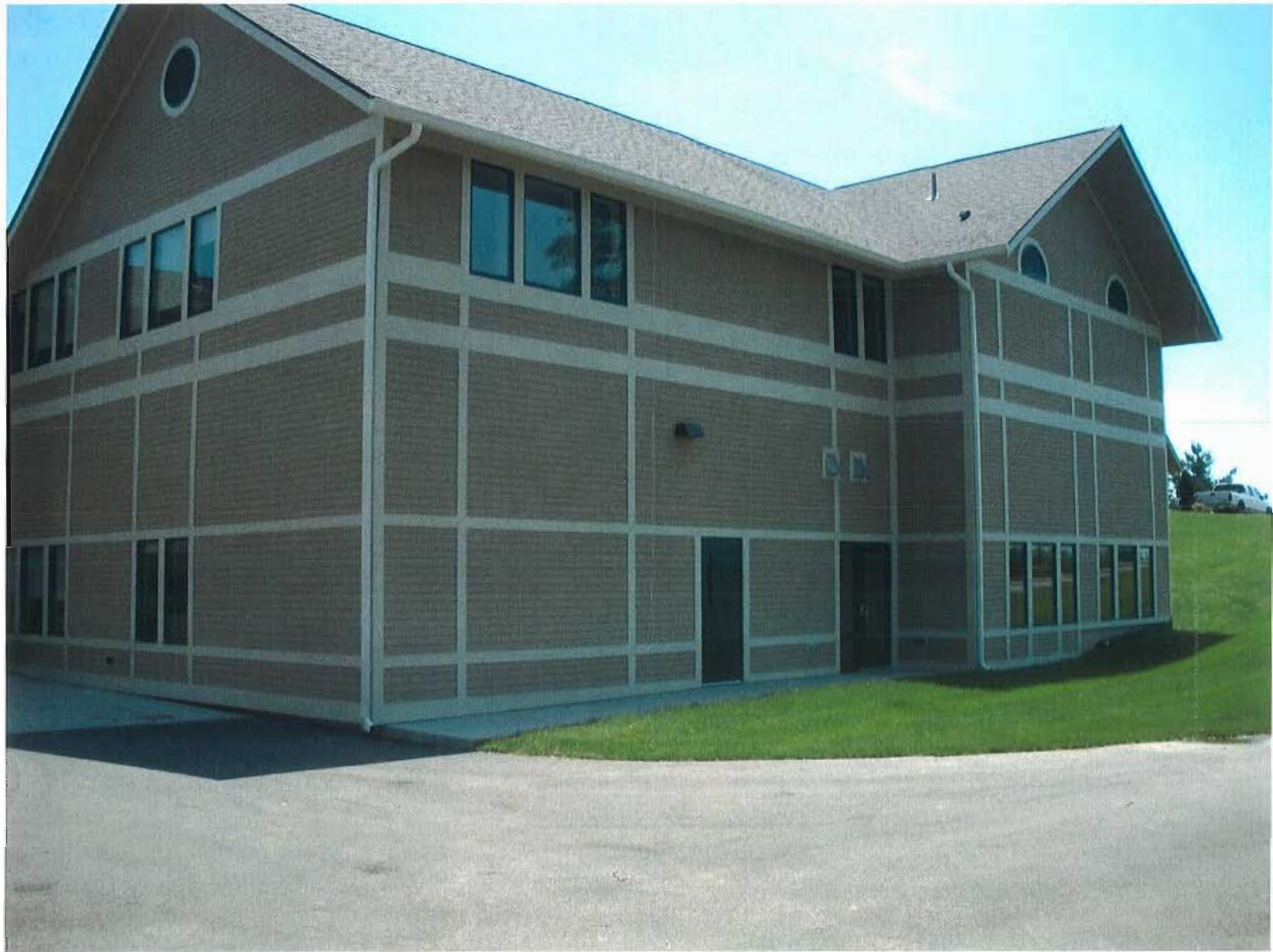
Existing View of West Elevation
