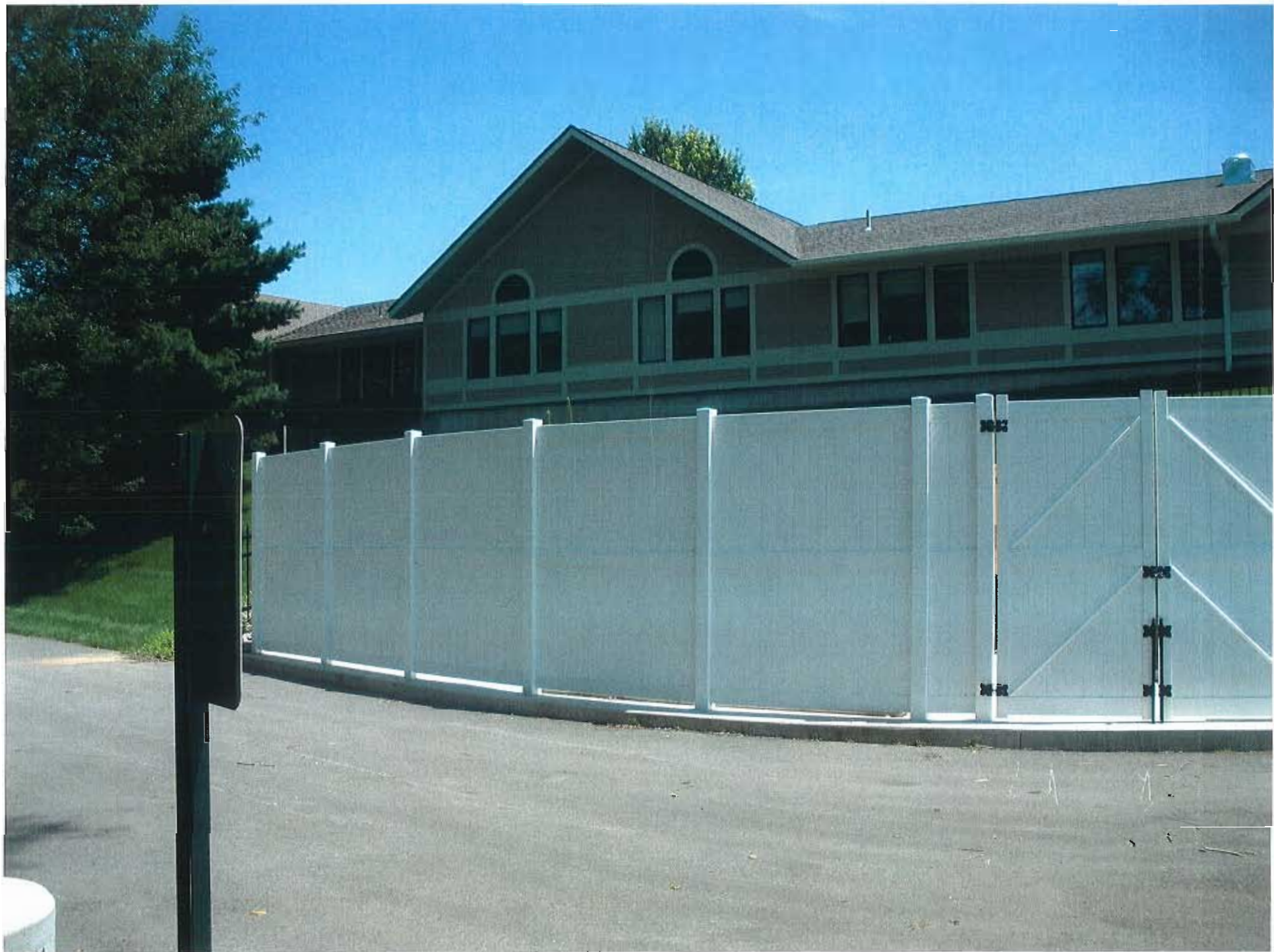
Existing View of West Elevation
