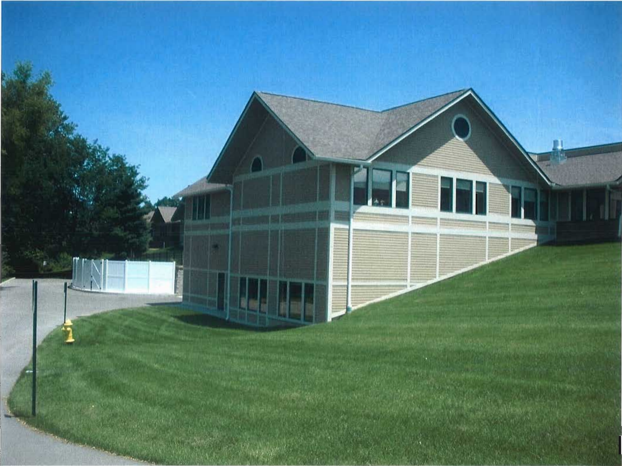
Existing View of South West Elevation
