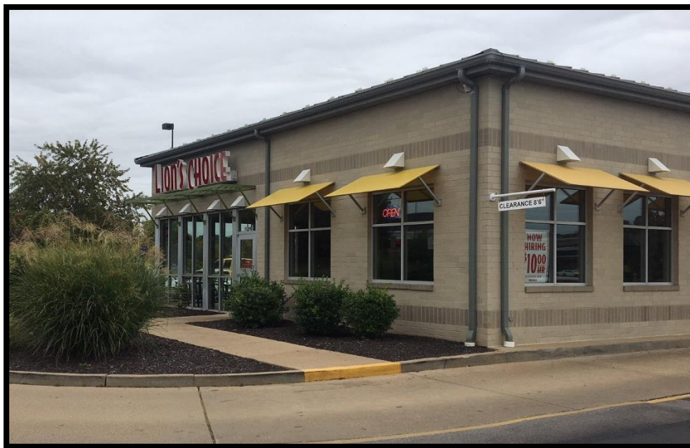
Figure 2: Existing Conditions of Northwest Corner
