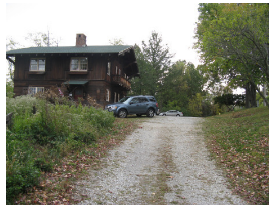
View looking south into the site
