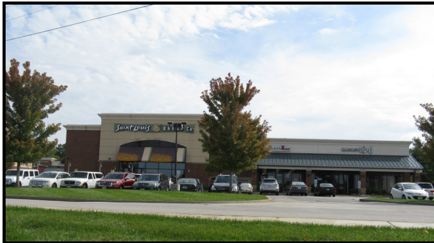
View looking east at the site.
