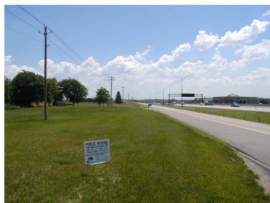
View looking east along N. Outer 40 Road
