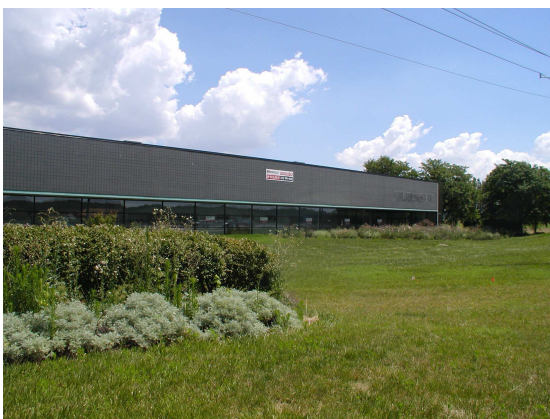
View looking north at the existing building.
