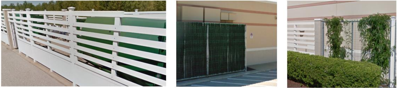
Figure 8: Existing Trash, Electrical Switchgear, and Utility Screening
