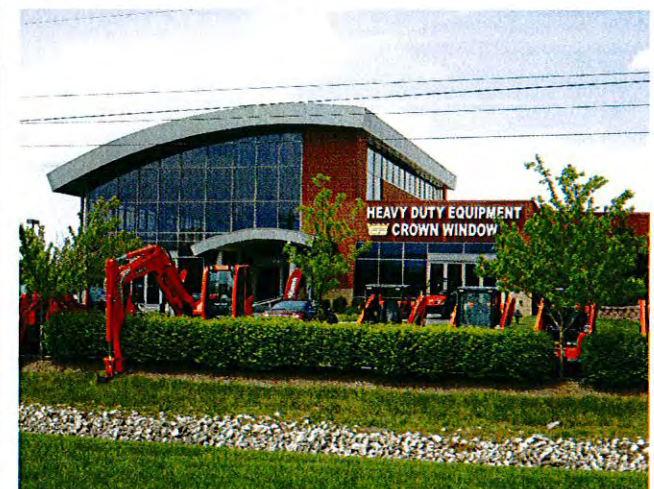
E - VIEW LOOKING NORTH (EXISTING BUILDING)
