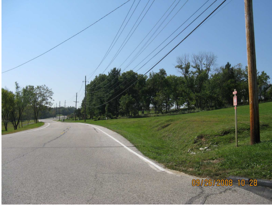
View looking south along the Outer Road
