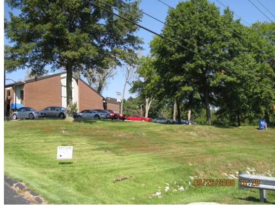
View looking into the property at the existing Church Building
