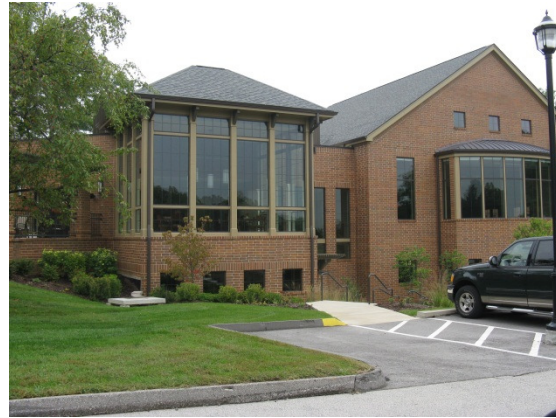
View of the Multi-Purpose addition
