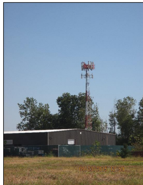
Figure 2: Photo of Tower
