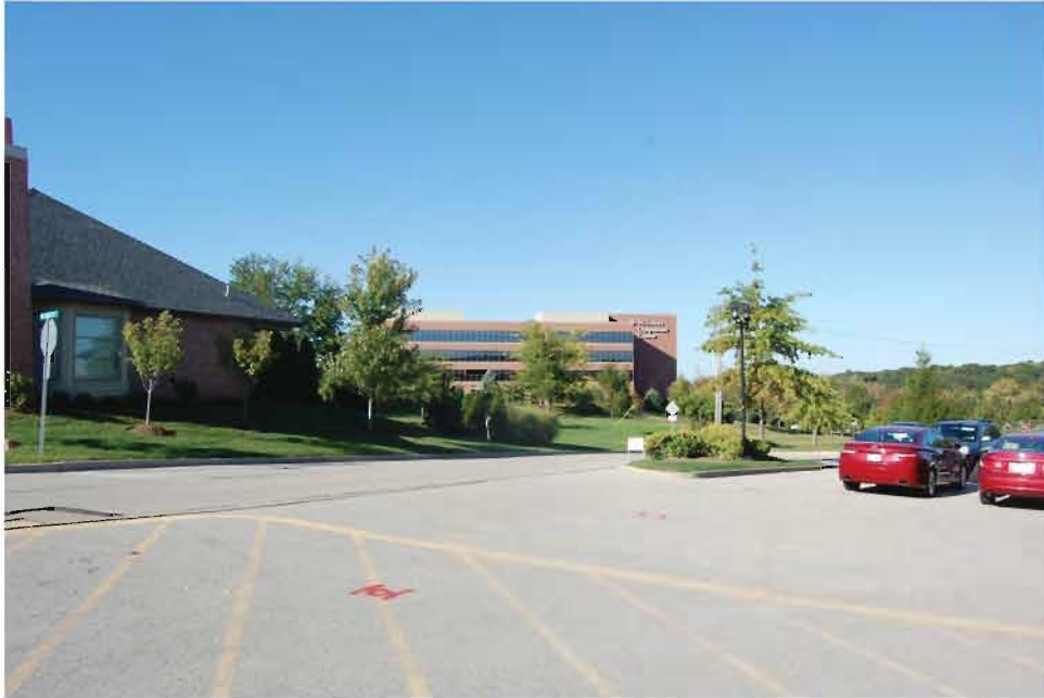
VIEW OF ADJACENT USE A - ST. LUKE'S HOSPITAL
