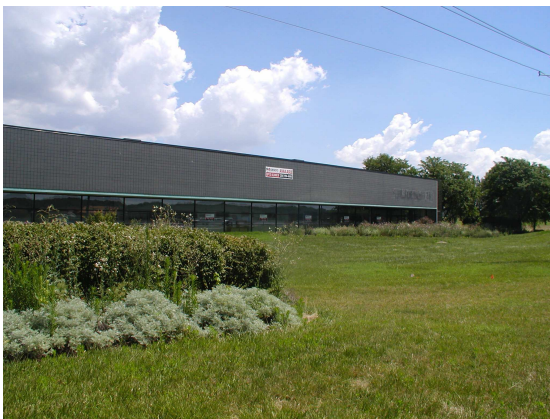
View looking north at the existing building.
