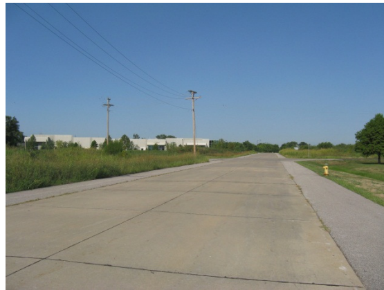
View looking west down Long Rd. Crossing Drive
