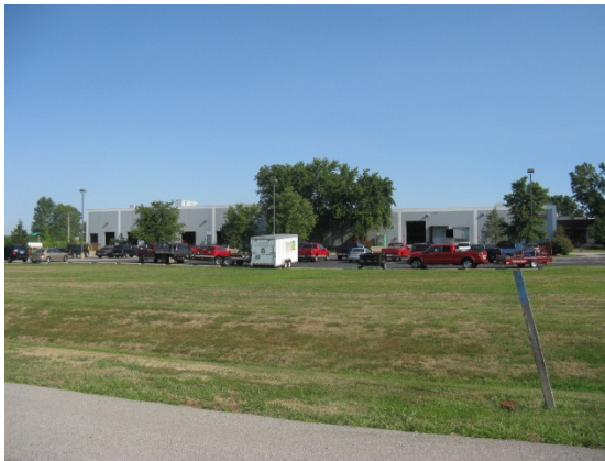
View looking north at the Cambridge Engineering building.
