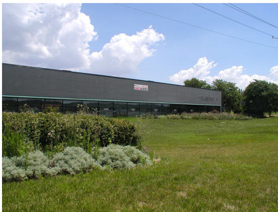
View looking north at the existing building.
