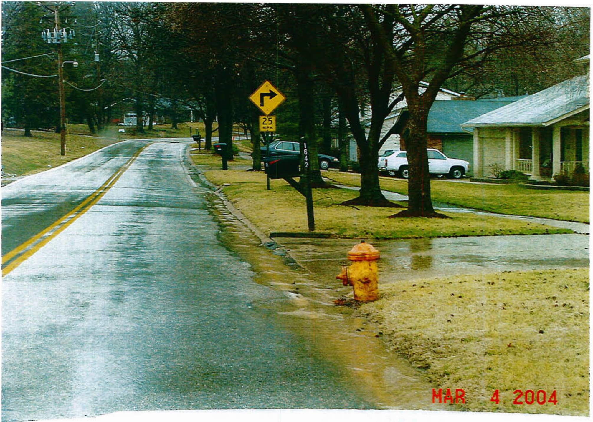
Old Baxter - looking north - showing east gutter line.JPG
