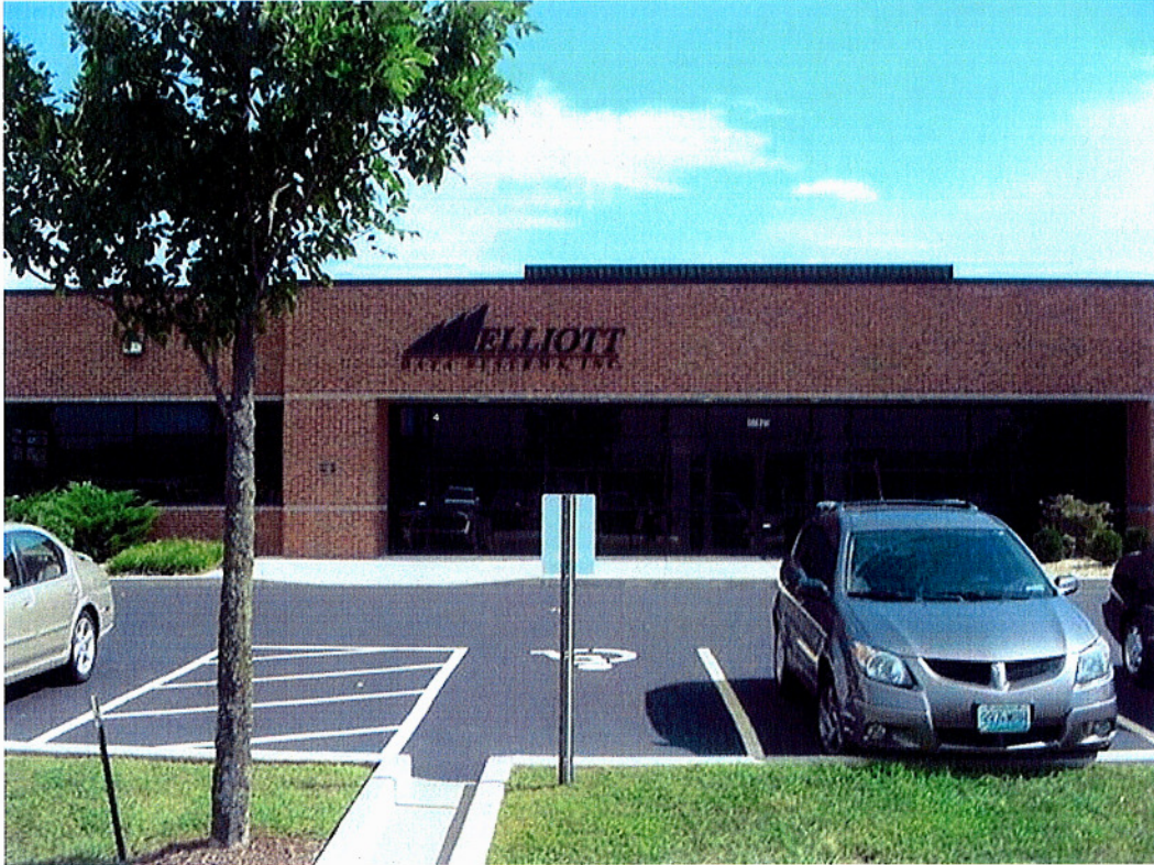
Figure 1: Existing Elliott Data Frontage as Seen From Edison Avenue
