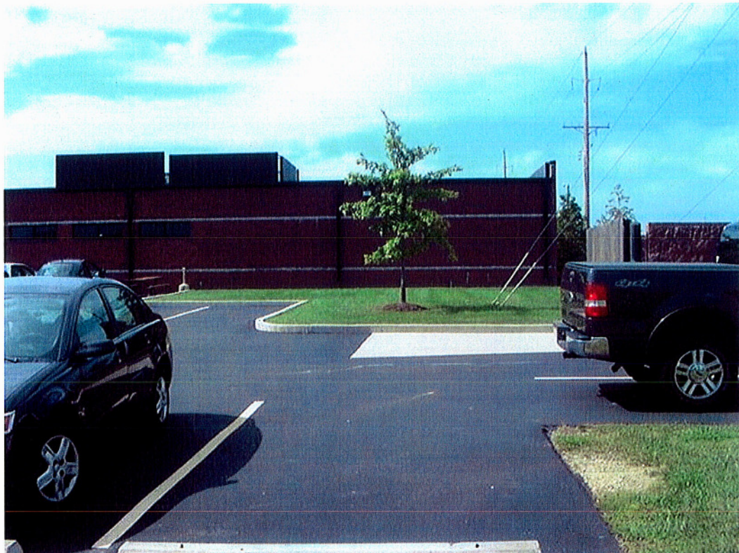
Figure 6: View from North
