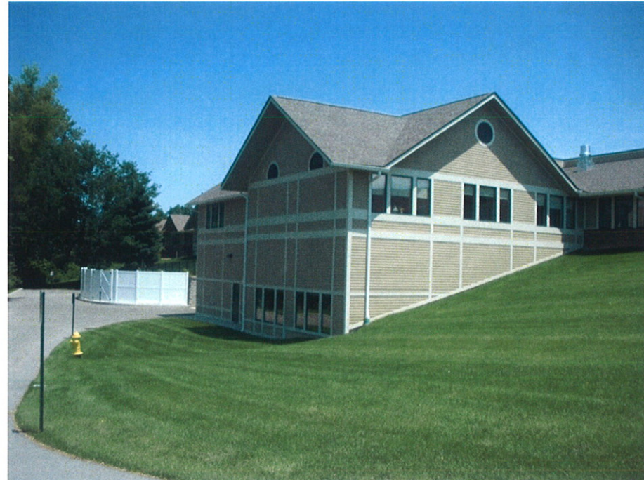
Existing View of South West Elevation
