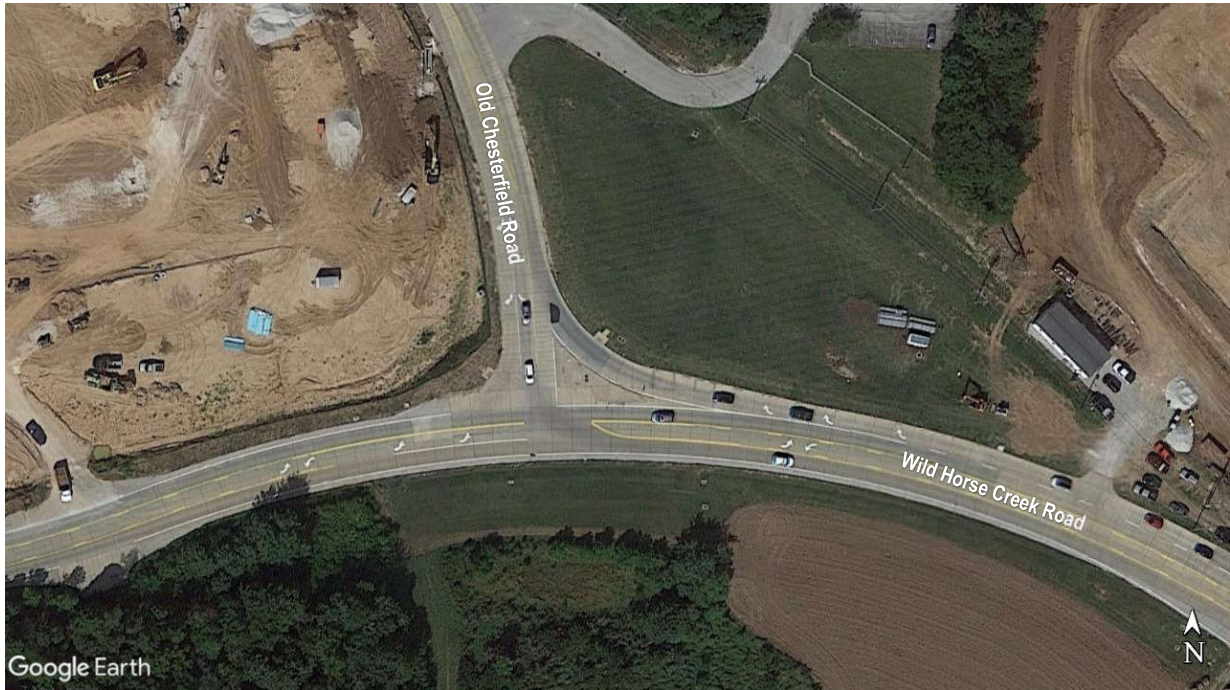
Figure 5: Aerial View of the Wild Horse Creek Road and Old Chesterfield Road Intersection
